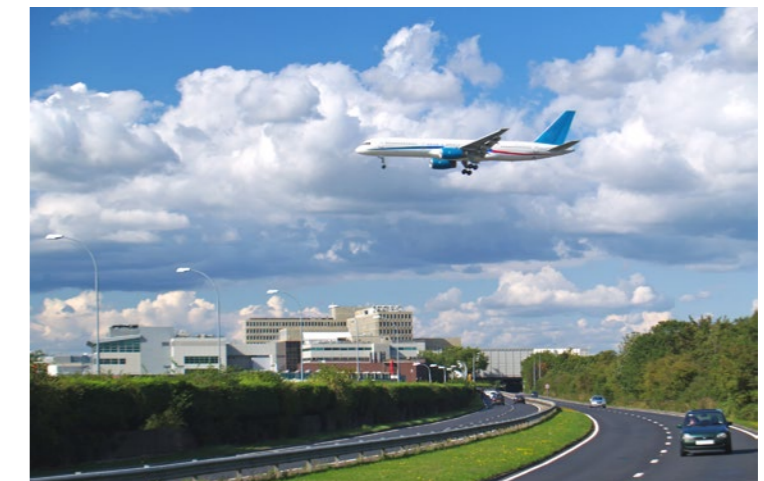
Figure 43. Gatwick Airport. South Terminal and Road Tunnel
